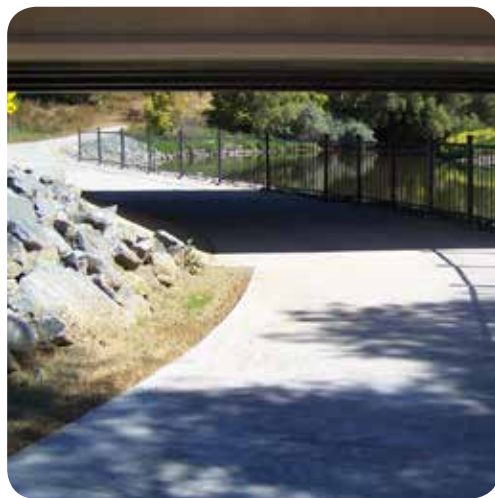
A new 0.9-mile section of the Poudre River Trail meanders along the Cache la Poudre River by the Swetsville Zoo and under County Road 5. Photo © Jeffrey Boring
