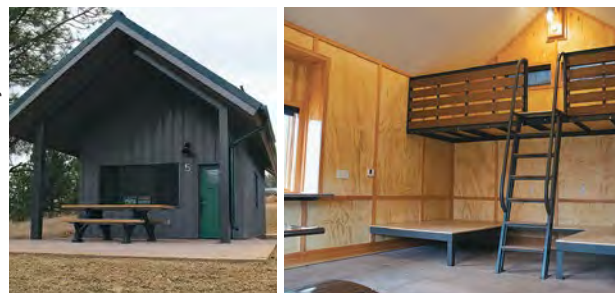
Five new camper cabins were built at Horsetooth Reservoir in 2021.
