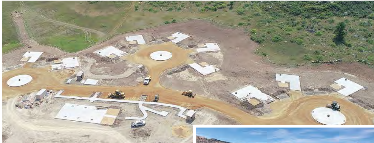
Aerial view of Sky View Campground during construction.
